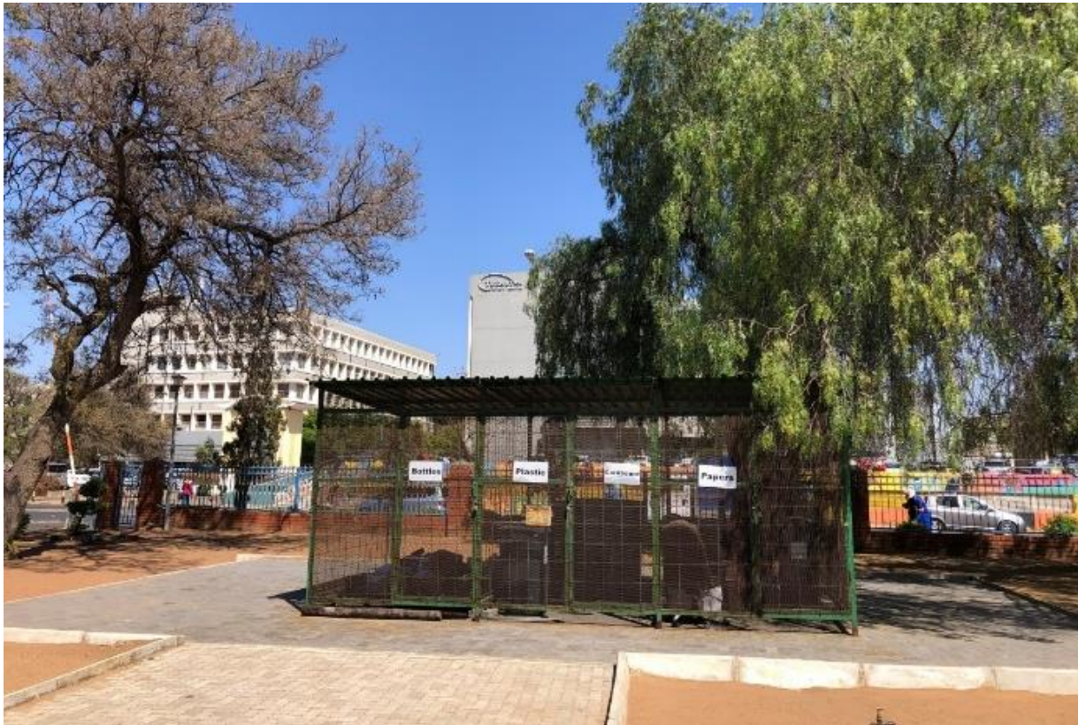
Recycling Station in Gaborone (Source: JICA Botswana Office)
