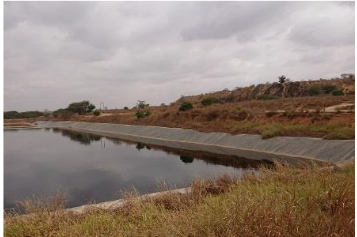
Leachate Treatment Facility
