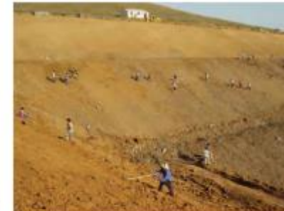
Slope forming before sheeting (2002)
