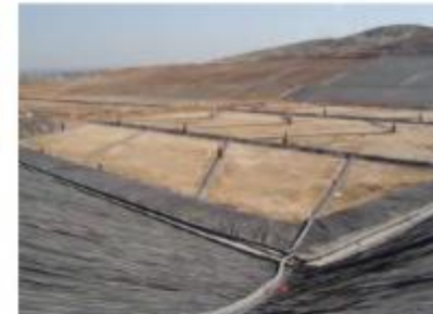
Completed landfill site(2003)
